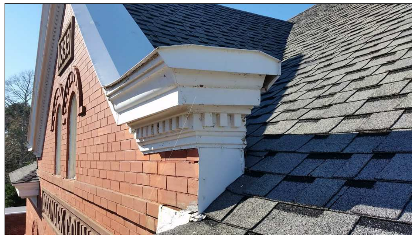
2 TYPICAL FLASHING AND COUNTERFLASHING TO BE REMOVED AND REPLACED
