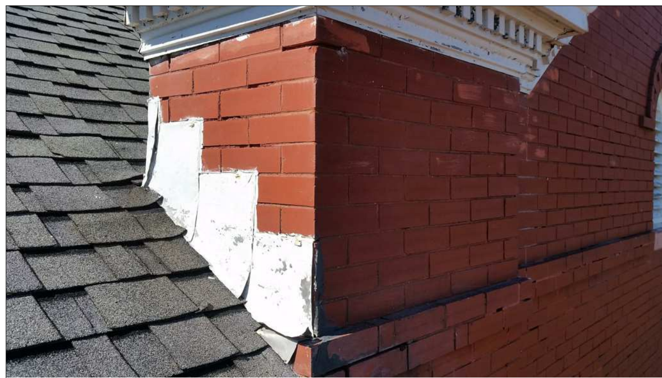
1 TYPICAL FLASHING AND COUNTERFLASHING TO BE REMOVED AND REPLACED
