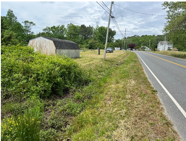
Roadside ditch looking west along Saxis Road.
