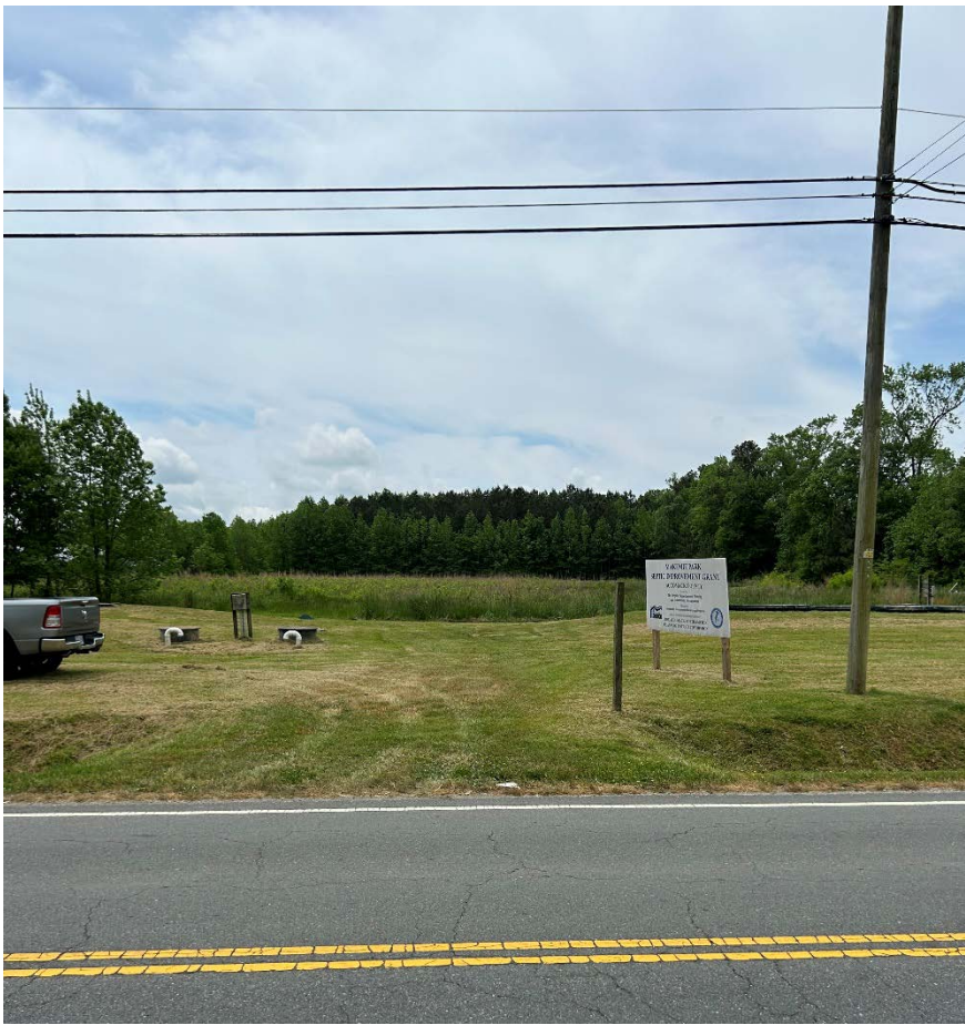
Entrance to facility looking south from Saxis Road. Pipe culvert below entrance connecting ditch on both sides.
