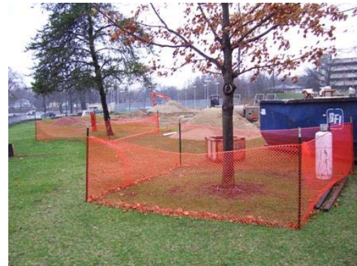
Improper (Above) and Proper (Below) Tree Preservation During Construction. Image Sources: National Tree Preservation and Elkhart County Soil and Water Conservation District.
