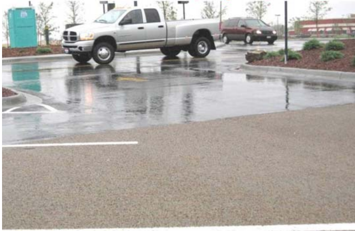
Above: Example of rainfall simultaneously on standard pavement (background) and pervious concrete (foreground). Image Source: Environmental Protection Agency
