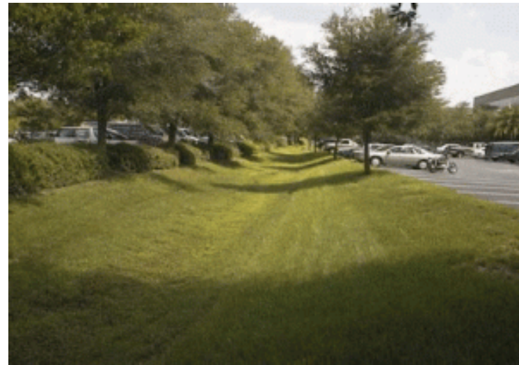
Above: Flow from parking area passes through filter strip prior to entering dry swale. Image Source: Virginia Department of Conservation and Recreation
