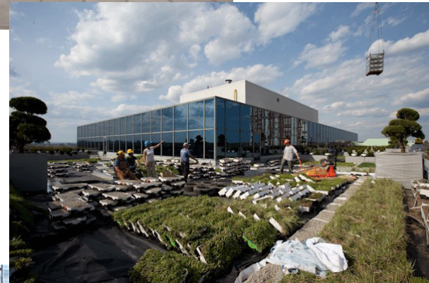
Top/Middle/Bottom: Example of an existing building in Toronto being retrofitted for a green roof with a combination of both intensive and extensive plantings with preplanted modular components. Image Source: Josephine Chan, ESRI Canada
