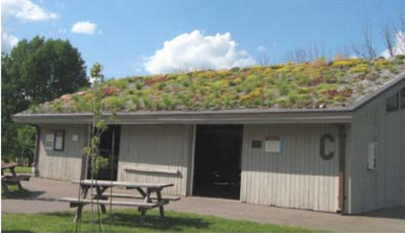
Above: Green roofs are not limited to flat roofs as shown in this example. Image Source University of Minnesota.
